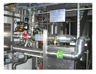
The heart of the system is the innovative MAKLAD INJECTOR. It is responsible for the heating of the wastewater to its inactivation temperature, and for cell disintegration. Additional main components of the System are the heat exchanger for preheating and cooling of the wastewater, the temperature holding tube, the wastewater pump, and the preheating vessel.
